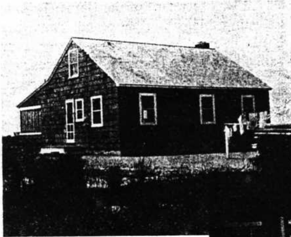
Original shore house before addition. (early 50's).
